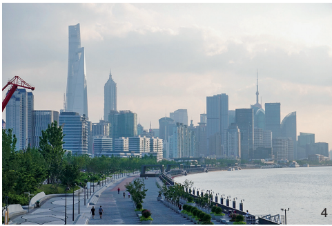
4 新华滨江绿地高桩码头 High-piled wharf in the Xinhua Waterfront
