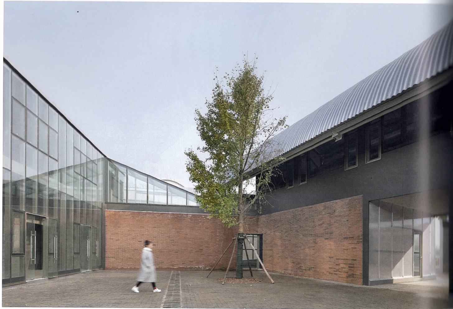
Contrast of various materials, including glass curtain wall, red brick, dark-gray steel panel, and silver corrugated steel panel
