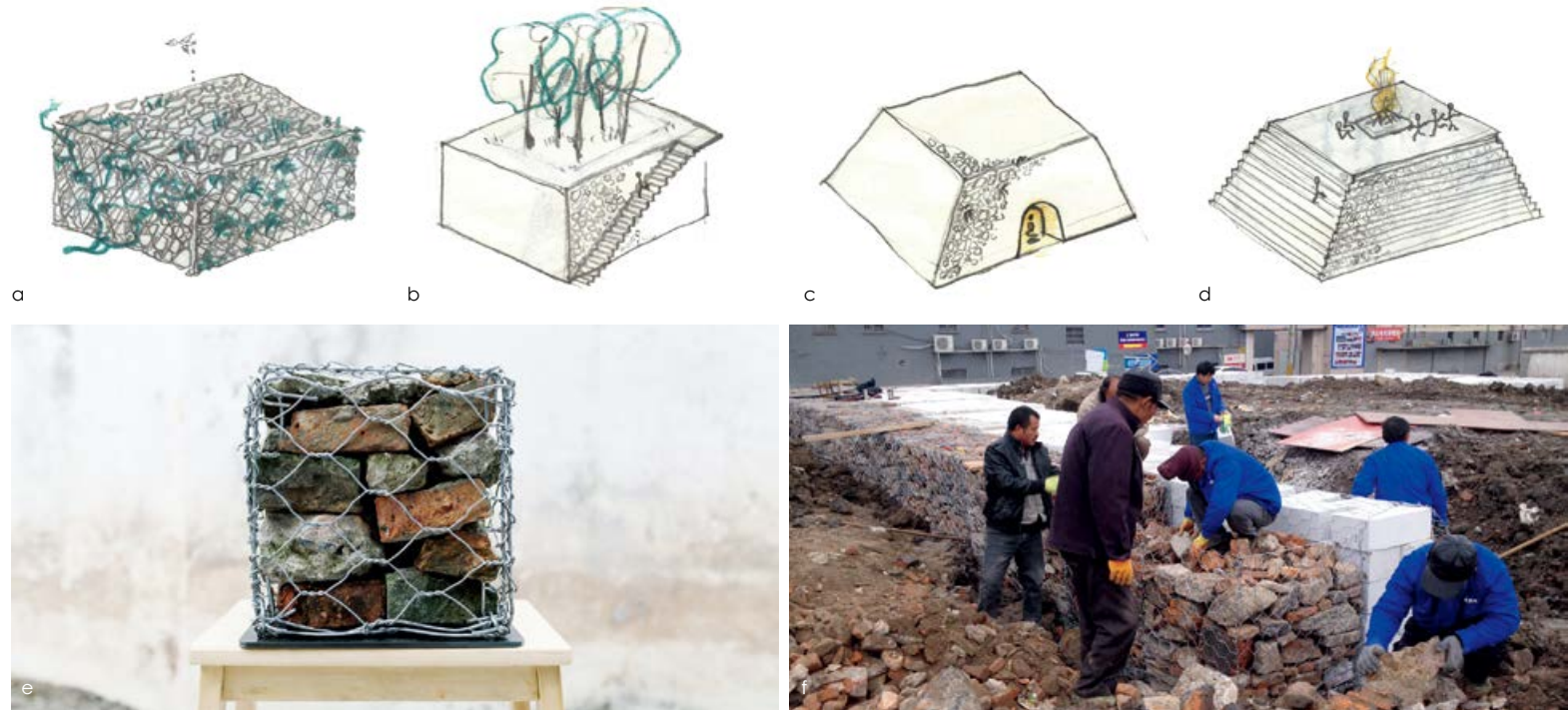
图3 / Figure 3 石笼构筑物 a,b,c,d. 石笼构筑物及石笼墙概念草图；e. 石笼模型；f. 石笼施工过程 Isometric of the gabions a,b,c,d. concept sketches of the gabions; e. gabion model; f. process of construction 来源：刘宇扬建筑事务所提供 / Source: Provided by Atelier Liu Yuyang Architects
